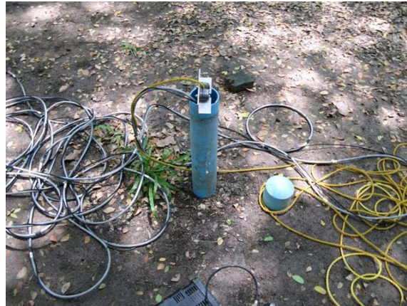
Figure 2.9 Make sure the geophone works. Then, put the geophone into the borehole and fix the safety rope with the holder
